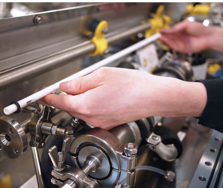
Ceramic membrane of the cross-flow membrane filtration plant
